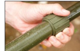
Rotate stem nuts and rinse again to ensure grit has been removed.
